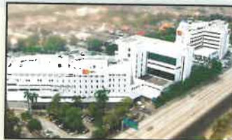
Sime Darby Medical Centre, Subang Jaya
