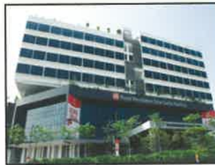
Desa Park Hospital
