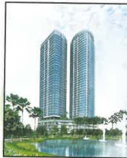
UOA Vertical Hotel, Bangsar South
